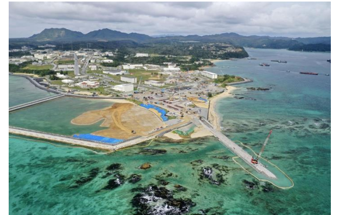
Henoko Marine Airfield Construction
